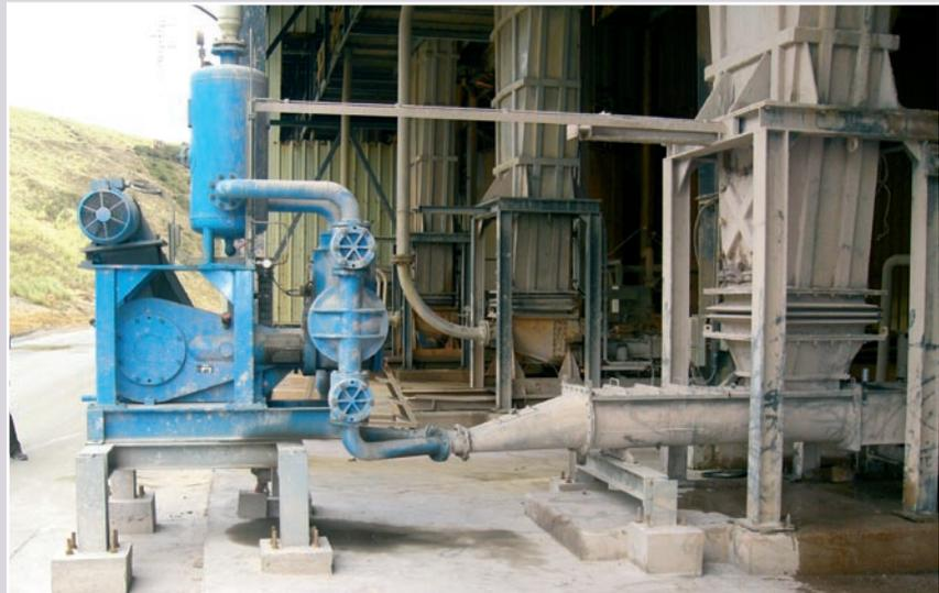
*Piston membrane pump type HMD-H-50-0500-ED with screw conveyor*
