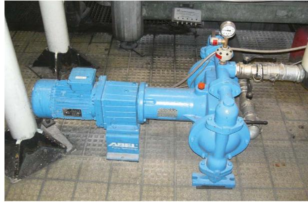
Electromechanical diaphragm pump, Type EM-040Z0300-SG as reflux pump for excess glue
