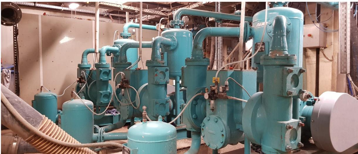
Hydraulic type HMD-G-32-0250 diaphragm pumps at GBAV
