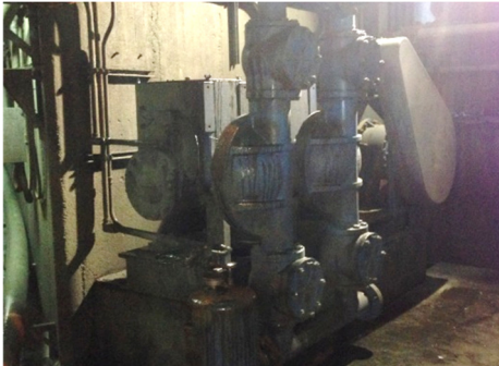
ABEL HM pumps: 70 m 3 /h and 6 bar pressure
